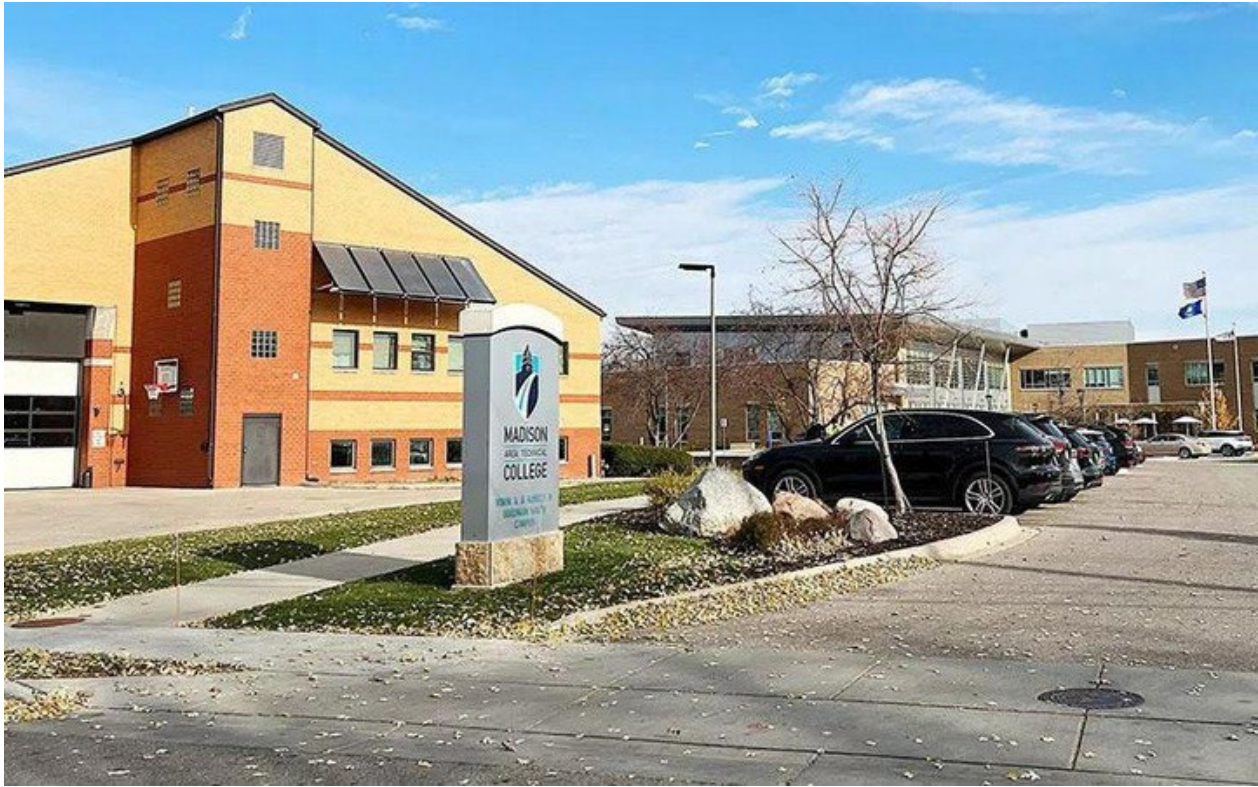
Fire Station No. 6 adjacent to Goodman South Campus
